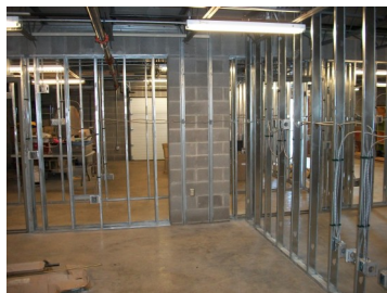
Basement with new framing for classrooms!
